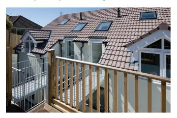
A four unit apartment block in an in-fill site. Built using the Thin-Joint method and large format aircrete blocks.
