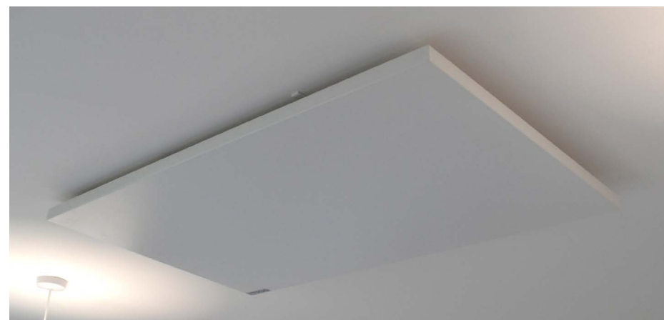
Infrared heating panel. Image provided by: Wondrwall.
