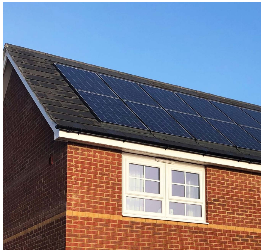
Photovoltaics can be integrated with the roof. Image provided by: Viridian Solar.
